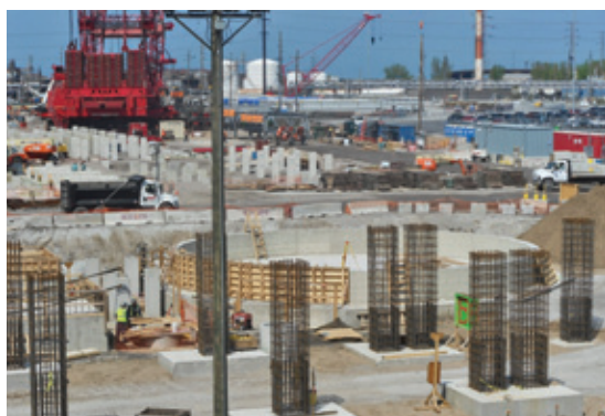
BIG POUR Baker contracted to pour 46,600 cu yd of concrete to accommodate a six-drum coker at a BP refinery in Whiting, Ind.
